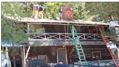
Repair of Chalet roof
